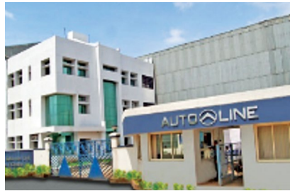
Unit 1 - Chakan, Pune, Maharashtra (Area - 11,400 sqm)
